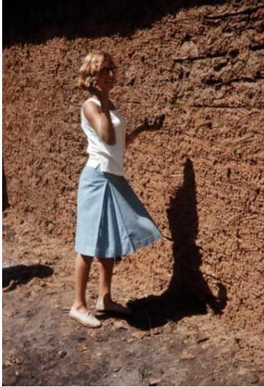
Janice working on the wall (7)
