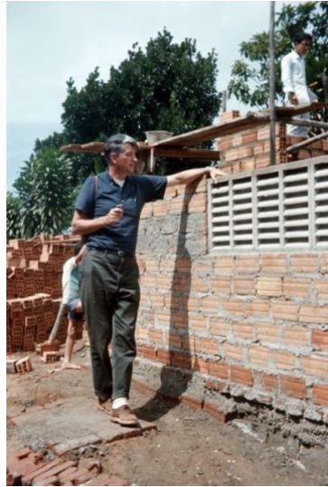
Bill Rogers inspecting our progress (8)
